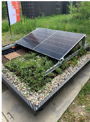
Figure 1: A photo captured during our visit to The Green Village showing a solar energy system that is designed to move to allow sun to reach the plants below it.
