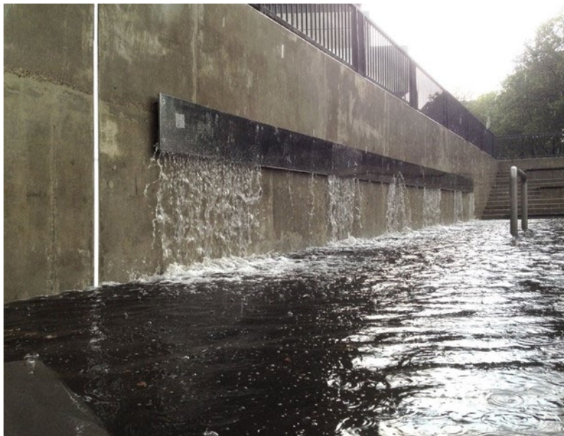
Figure 7. Water flowing into a basin during heavy rain in Rotterdam. Photo by Jurgen Bals ( https://www.urbanisten.nl/work/benthemplein ).
