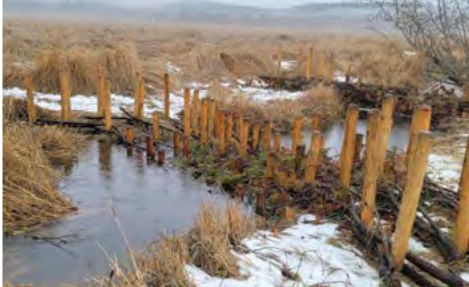
This photo taken by Professor Niezgoda shows a completed starter dam in the foreground and a secondary dam behind it
