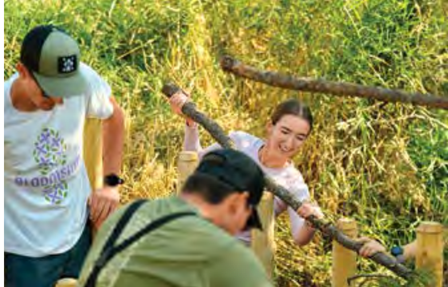
Students weave young pine boughs between posts, creating a textured fill that forms the core of the beaver dam analog
